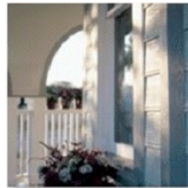
Door and Window Surrounds
