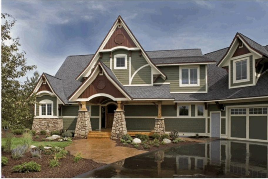
James Hardie lap and shingle siding with ColorPlus® Technology featured in MidWest Homes' Minnesota Top Homes Volume 2 . The home was built by Mark Anthony Homes in Hudson, Wisconsin.
