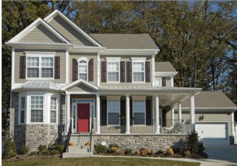
This house in Nashville, Tennessee, features HardiePlank™ lap siding in the ColorPlus® Technology colour, Woodland Cream, with HardieShingle™ siding in Woodland Cream and HardieTrim™ boards in Arctic White.
