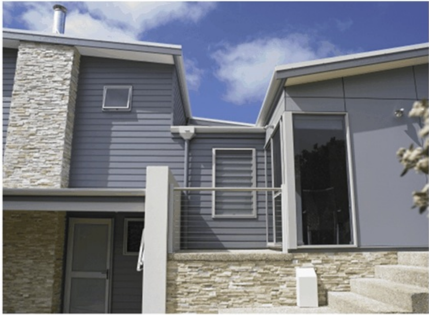
Holiday house in Western Australia with PrimeLine weatherboards and Scyon™ Matrix cladding.
