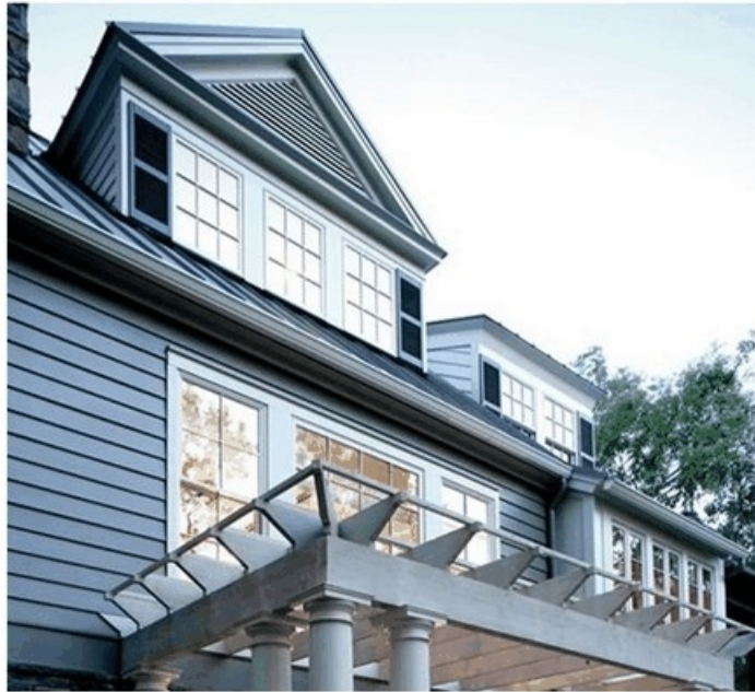
Architect John Tee and builder John O Freeman Jr selected Artisan® Lap for the Southern Living Idea House at Reynolds Plantation, Greensboro, Georgia
