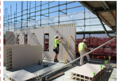
Permanent Form Work
