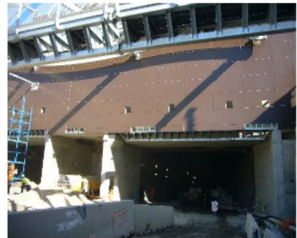
NSBP Tunnel Brisbane, Australia
