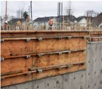
Temporary Formwork
