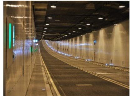
Elbe Tunnel Hamburg, Germany
