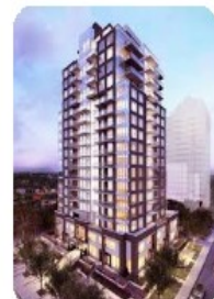
Ultra High Density ( >12 Storey)
