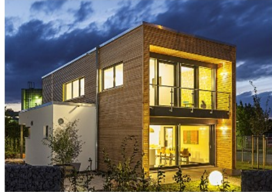
New timber frame home in Hameln, Germany
