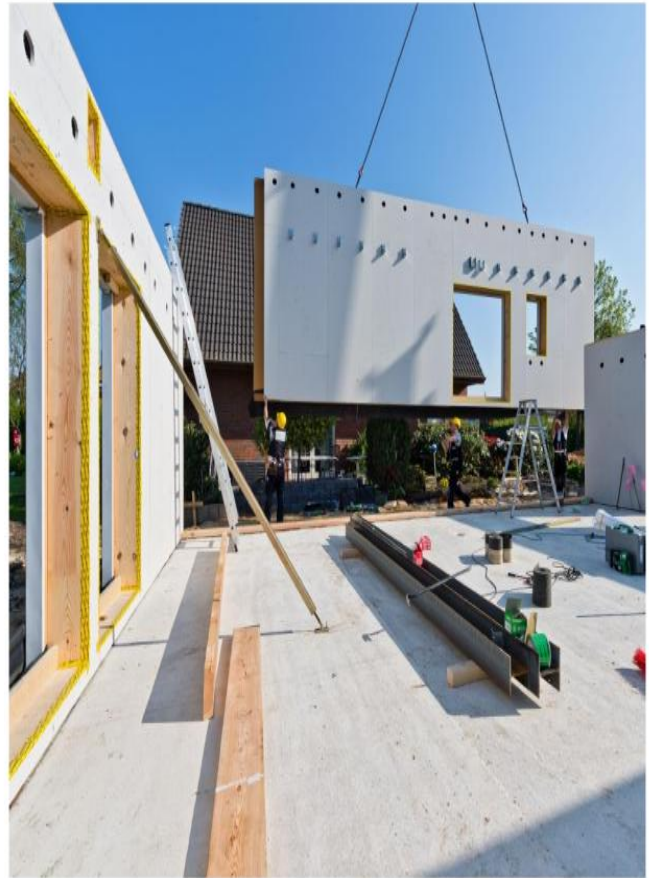
Pre-fabrication construction in Germany
