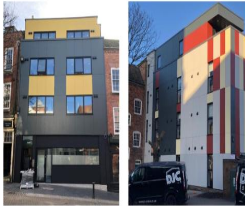
Hardie® Architectural Panel project (Worcester, UK)
