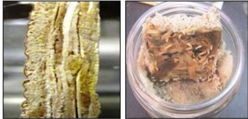
Mold Growth Termite Activity
